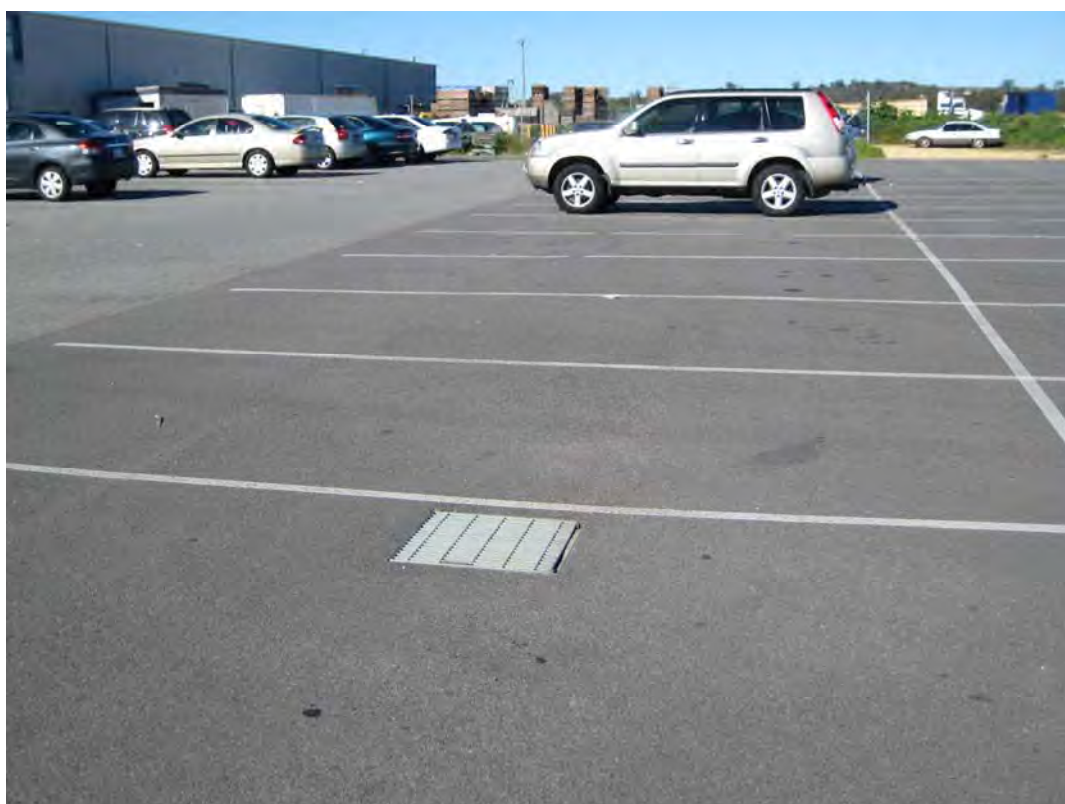
PLATE 8 – Stormwater drains located in the car park on Lot 299 Kerosene Lane, Baldivis.
