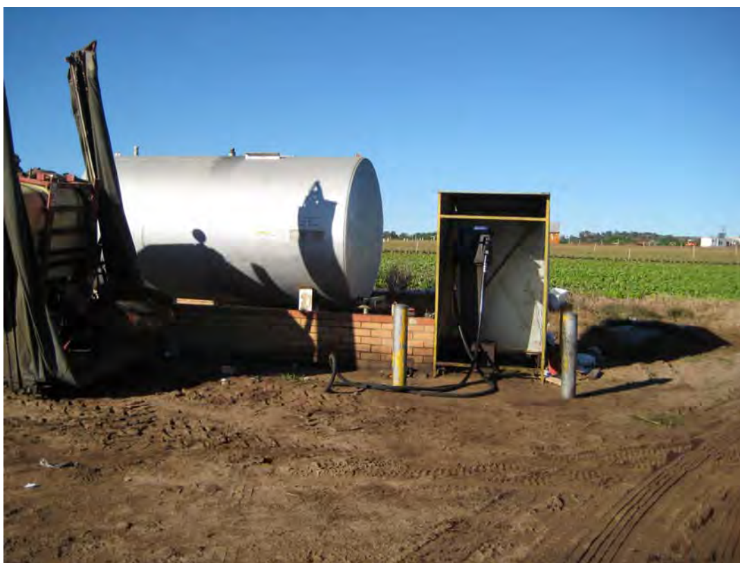
PLATE 1 – Fuel storage area.
