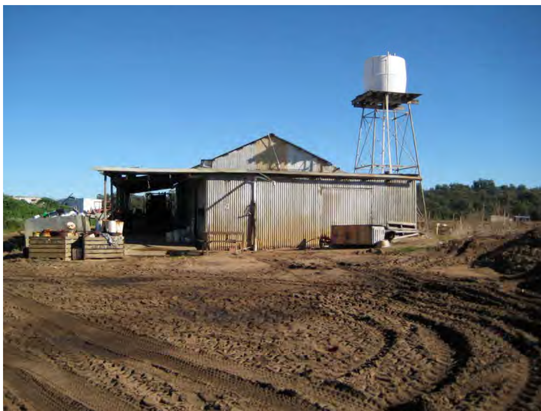
PLATE 4 – Chemical shed on Lot 14 Kerosene Lane, Baldivis.
