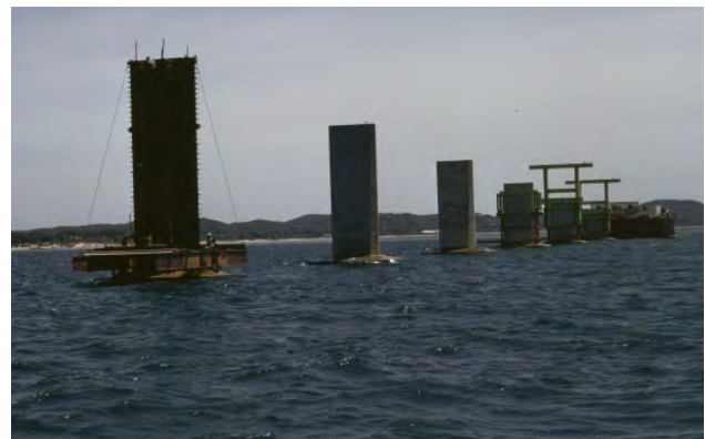
Image 83: Construction of the Causeway
