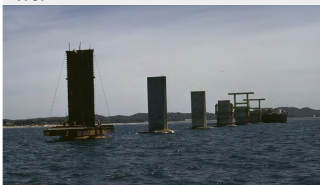
Garden Island naval facility was announced by the Australian Government.
