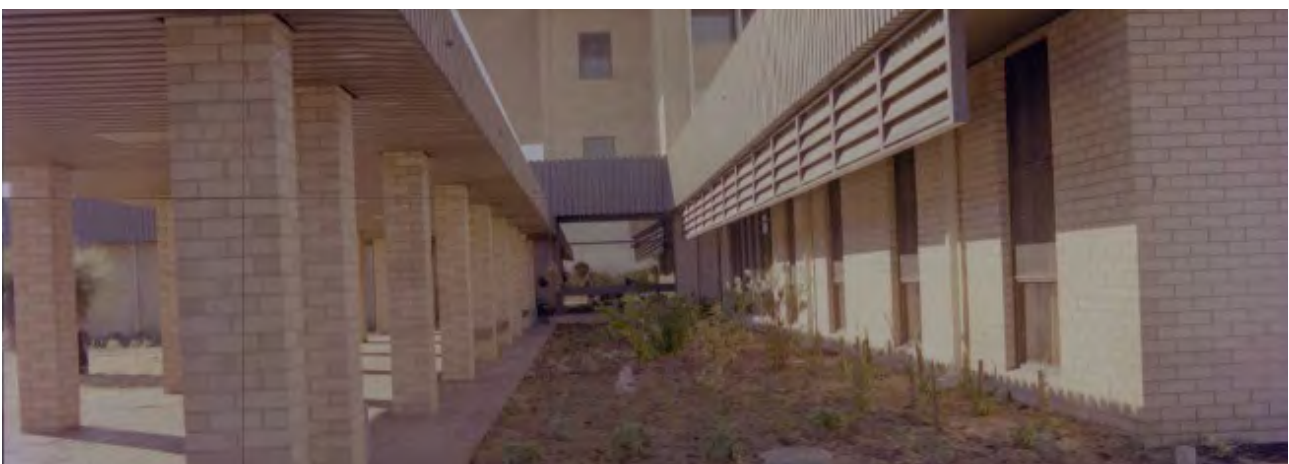
Image 84: Construction of the District Hospital
