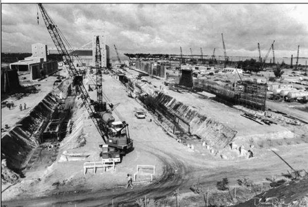
Source: Construction of Kwinana Grain Terminal, 1969. Courtesy of Joan Hartley Pitchard in History of Rockingham Kwinana Facebook Group.
