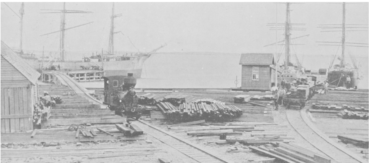
Image 59: Timber Jetty at Rockingham Beach
