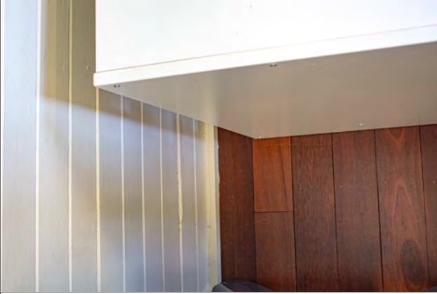
skirting and timber hardwood, building 1
