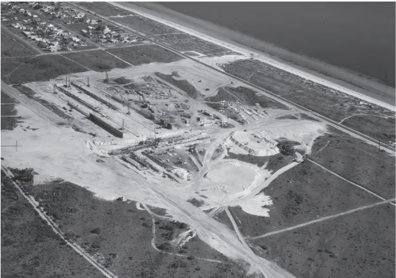
Image 79: Construction of the Kwinana Grain Terminal
