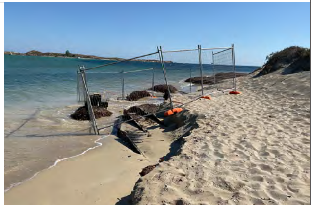
former jetty structure
