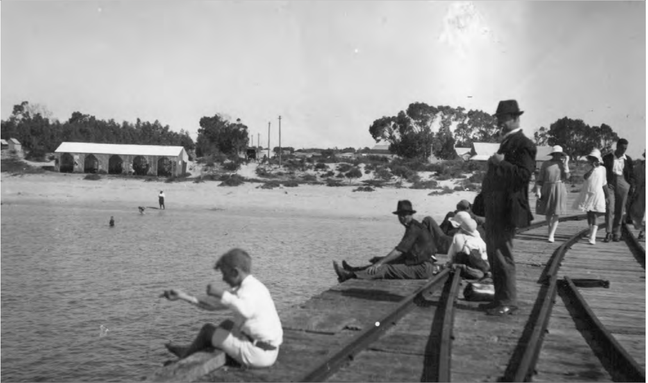
Source: '011974D: Jetty at Rockingham' State Library Western Australia, 1923.
