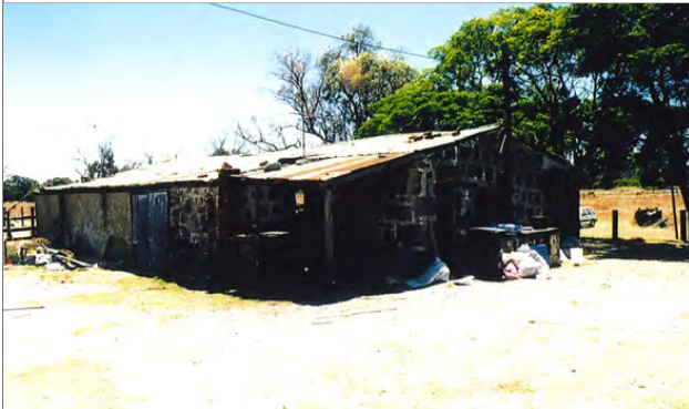
former dairy (demolished)
