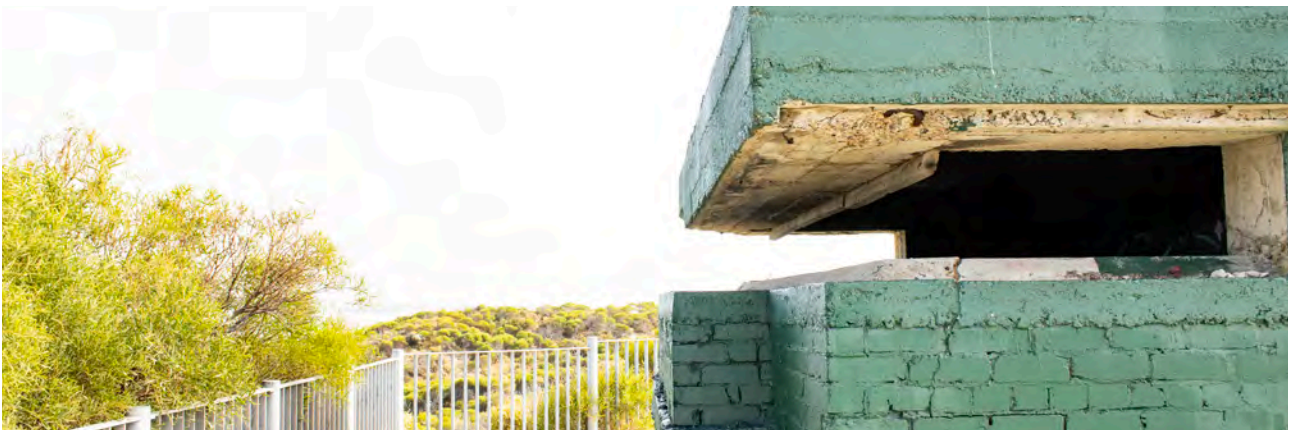
Image 9: State Listed Place, Cape Peron K Battery Complex
