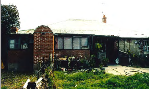
Hymus House prior to conservation works
