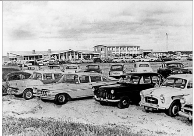
Source: the Rockingham Museum showing the Waikiki Hotel and its construction 1960.
