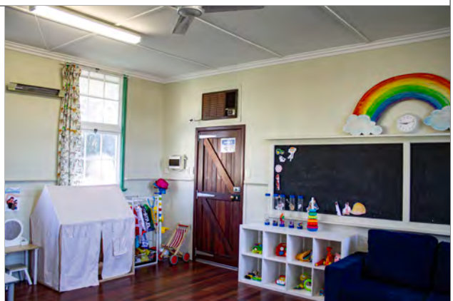
timber exit with chalkboard, building 1
