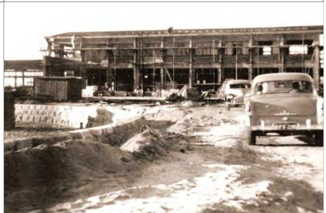
Source: the Rockingham Museum showing the Waikiki Hotel and its construction 1960.
