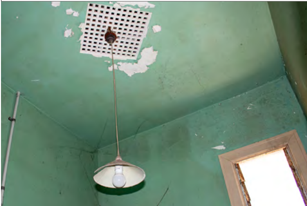
fitting in storage
