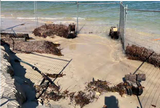
former jetty structure
