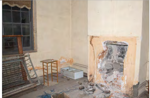
sash window and fireplace (no longer extant), R3
