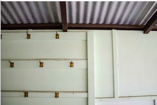
entry with bag hooks, building 1
