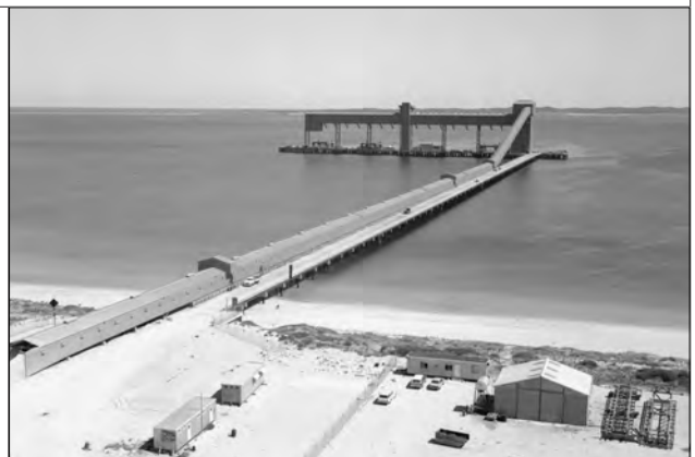
Source: Kwinana grain Terminal, Mark Hotchkin ,1976, SLWA
