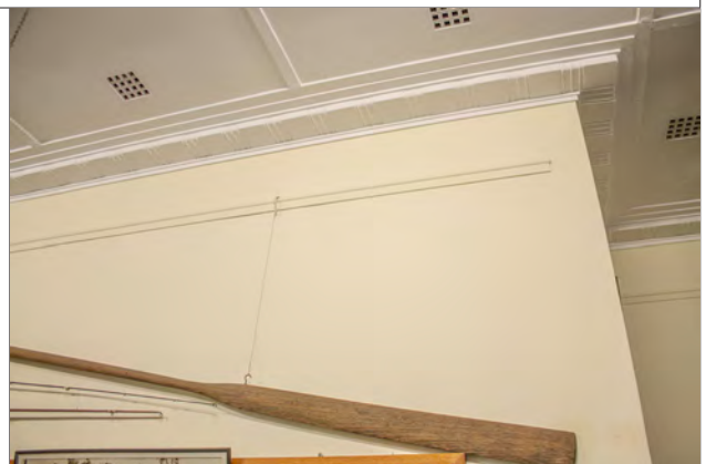
picture frame rail and moulding with catalpa oar
