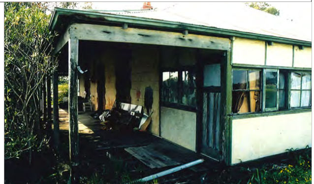
Hymus House prior to conservation works
