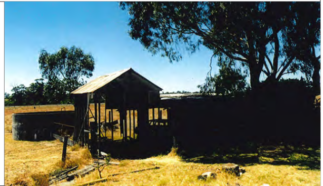
former outbuildings (demolished)
