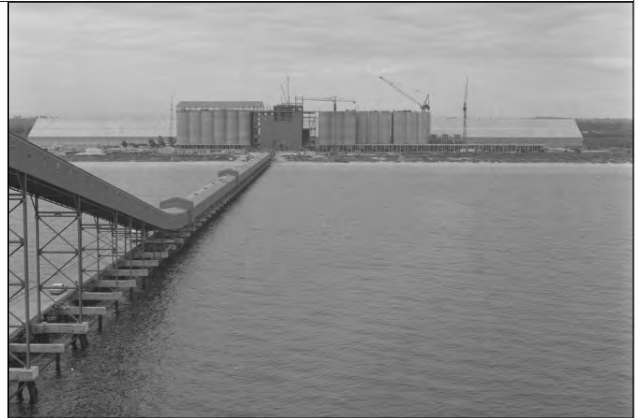
Source: Kwinana Grain Jetty under construction, 28 July 1975, SLWA, 361571PD
