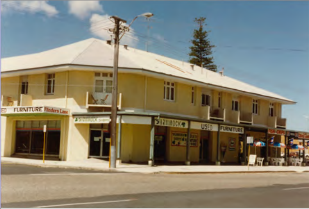
Source: 'Trocadero Dance Hall, West to Rockingham Beach Road, 1993' Rockingham Hotel Heritage Assessment, Ronald Bodycoat & Assoc Pty. Ltd., 1993.
