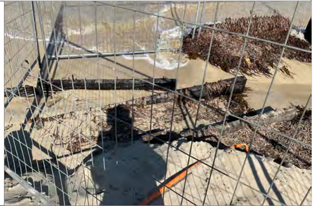
former jetty structure
