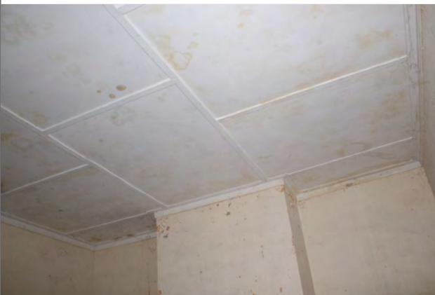
battened ceiling R3
