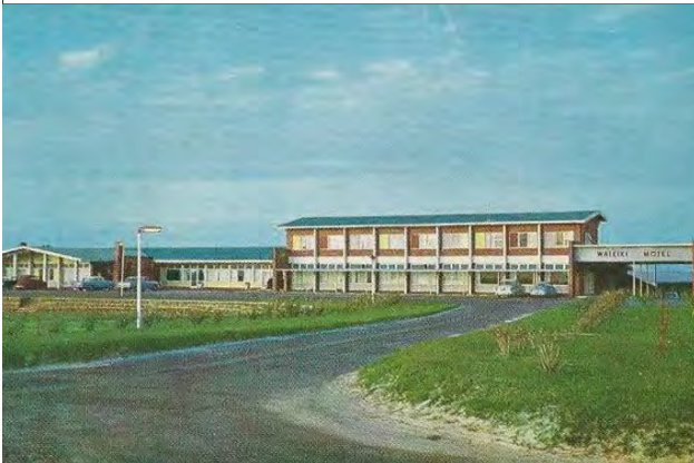
Source: the Rockingham Museum showing the Waikiki Hotel and its construction 1960.
