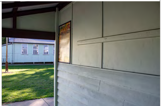
weatherboard and CFC cladding, building 1
