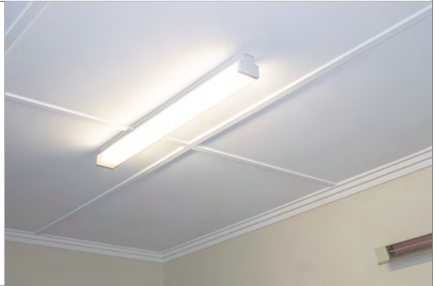
battened ceiling with lamp, building 1
