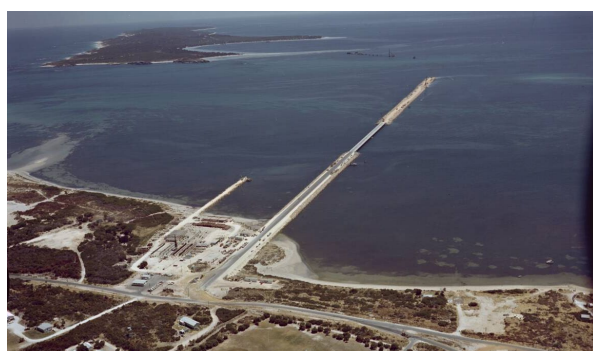
Figure 16 Source: Construction of the Kwinana Grain Terminal and Jetty, 1969 State Library of Western Australia. 262639PD
