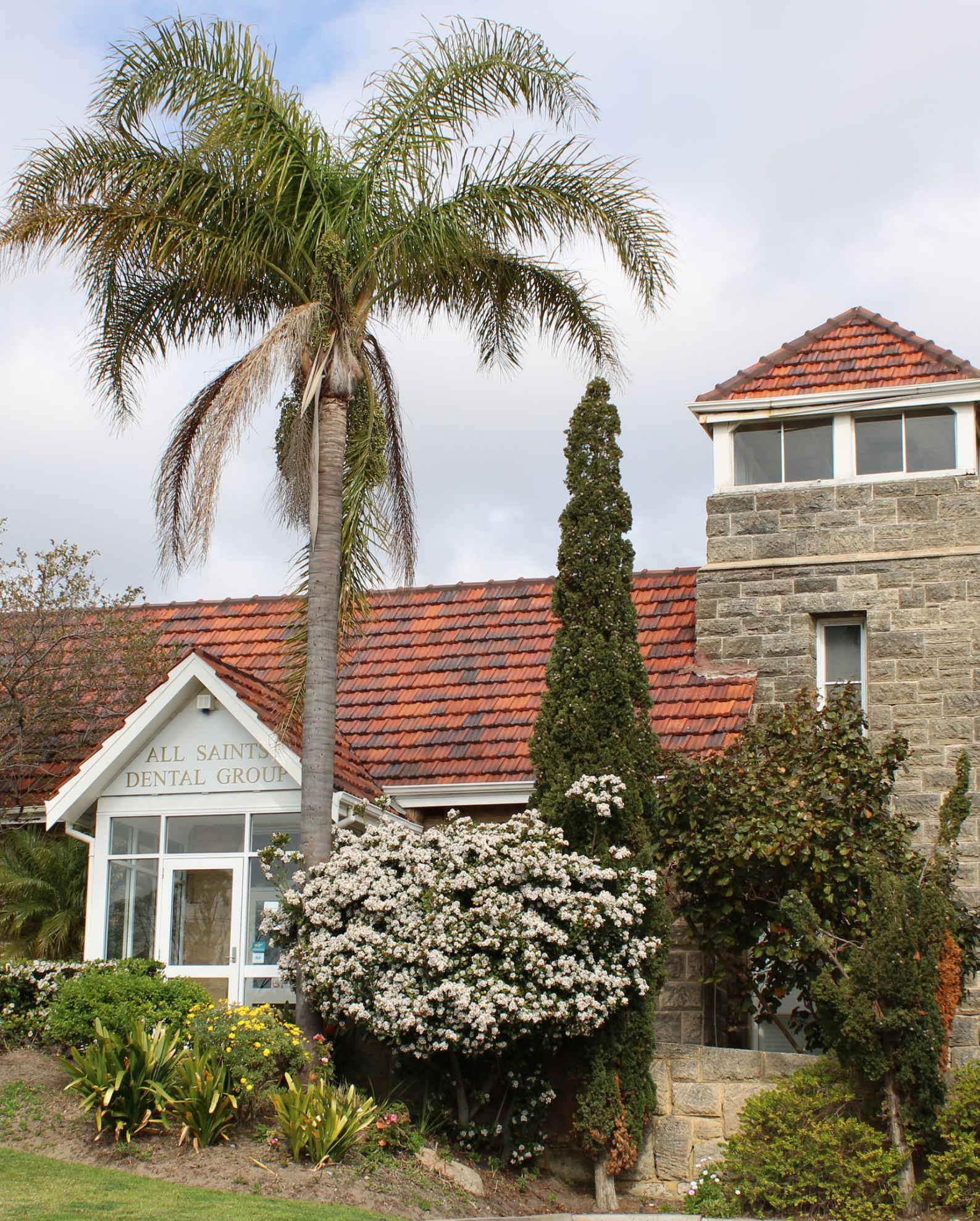
Anglican Church (fmr) built 1945 Building adaptation since 1990s
