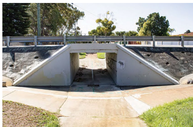
Figure 19 Rockingham Underpasses for the Rockingham Park Estate by Rockingham Park Pty Ltd from 1969 - Source: Murals by Paul Ritter, Stephen Carrick Architects, 2024
