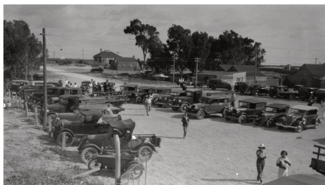
Figure 12 Rockingham Hotel Car Park source: 'Rockingham Hotel Carpark', 1935. State Library of Western Australia
